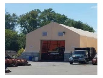
Constructed in 2014, this facility is 3,570 square feet and is used for equipment and vehicle storage. The building is a fabric membrane, stretched over a steel structure, with a v-block concrete foundation.
