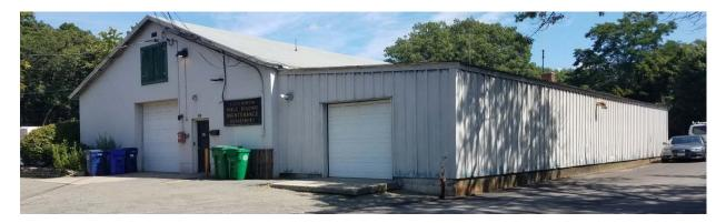
This building is 7,640 square feet. The building is comprised of a 3,780 square foot concrete block garage built in 1968, a 1,700 square foot metal prefab garage added in 1976, and a 2,160 square foot wood framed modular section added in 1980. This facility has 25 employees assigned to it, 12 of which have assigned offices that are heavily occupied. The other 13 employees are trades craftsmen who use the facility for work assignments and bathrooms.
