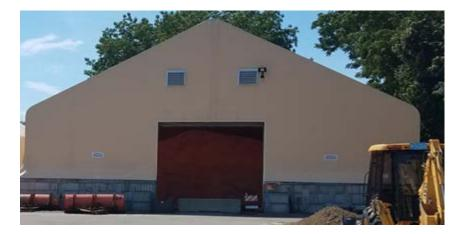
Constructed in 2014, this facility is 6,305 square feet and houses road salt for the north side of the City. The building is a fabric membrane, stretched over a steel structure, with a v-block concrete foundation.
