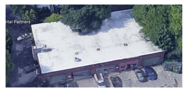
Built in 1959, and partially renovated in 1993, this 7,548 square foot cinder block slab on grade building houses mechanical repairs, storage, property and evidence, and support services.
