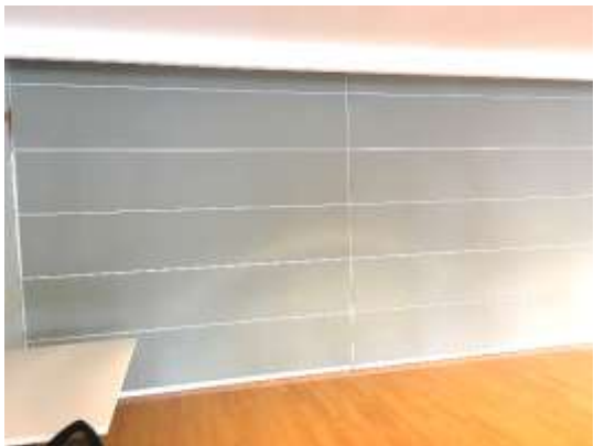
Automatic roll down dividing wall, more expensive but easier to use and takes up less floor space, needs space above ceiling when fully opened
