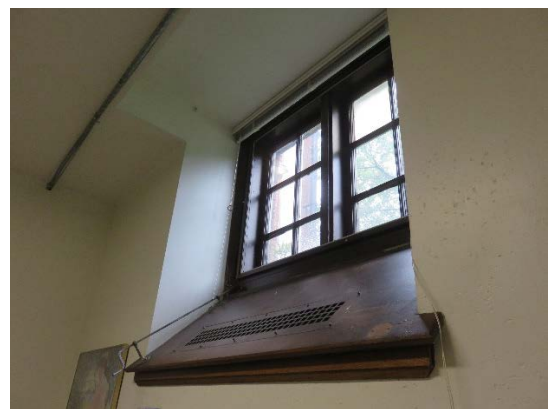
Original wood window sill with heat grille.
