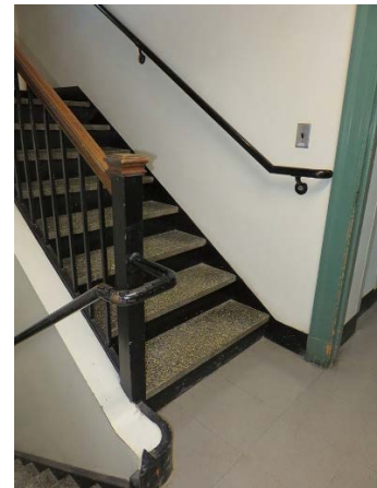
Added handrail at wall.
