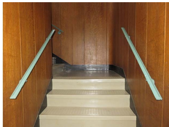
South stair at ground floor level has rubber treads.
