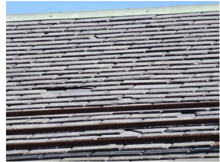
Missing and broken slates.
