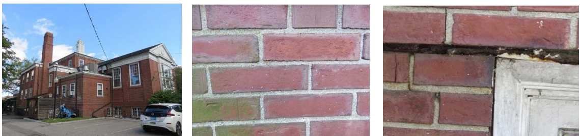
General view of brick, close-up, and detail showing deteriorated mortar joints and rusted lintels.
