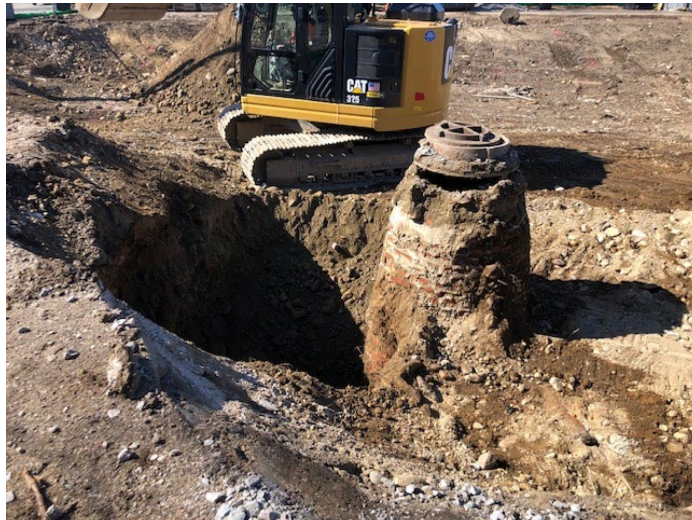
Removing Existing Sewer Manhole
